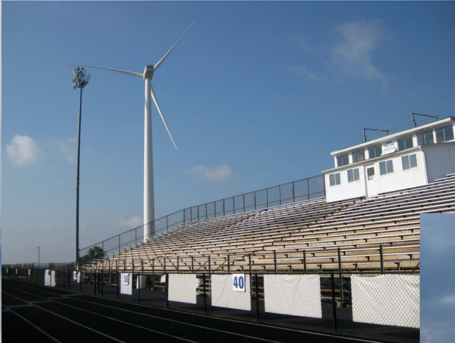
Turbine in fully feathered brake position in front of an empty stadium
